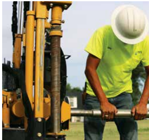
Left: PTCI Heavy Equipment Operator Billy Perez places a beacon into the head of the boring machine. The beacon communicates from below ground to the locator above ground to know which direction the boring head is going both vertically and horizontally.
